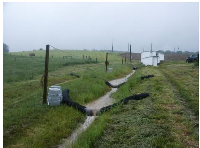
*Downstream of a gauging station at NAEW during a runoff event.*
