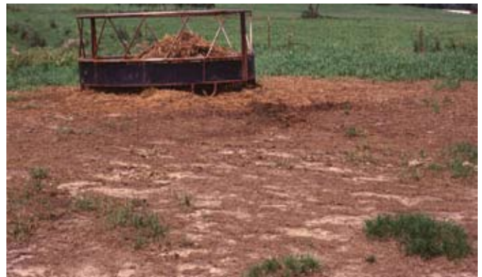
Heavy use areas, such as around this feed bunk, often wash during heavy rains. Note missing hay residue at the bare spots in foreground.
